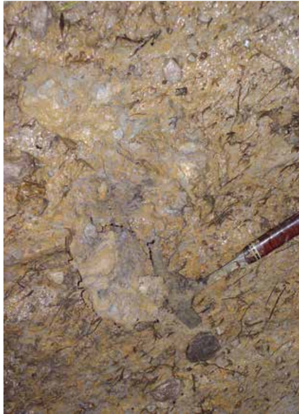
Figure 5.2: Close-up of mottling in subsoil
